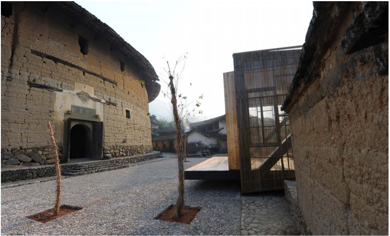
North entrance of the building, in front of the Hakka Castle.
