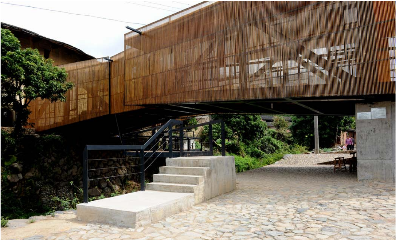
Access stairs to the hanging bridge over the river, from the west bank
