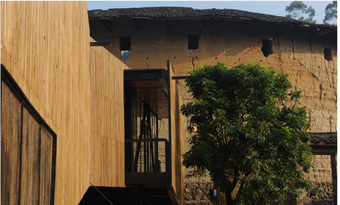
View of the corridor from outside.
