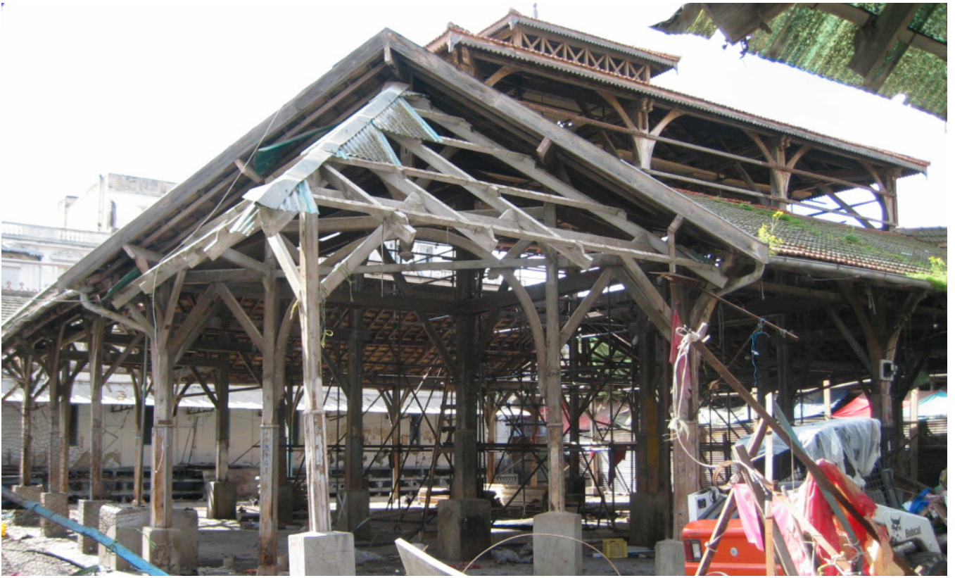
Central wooden covered market before restoration.
