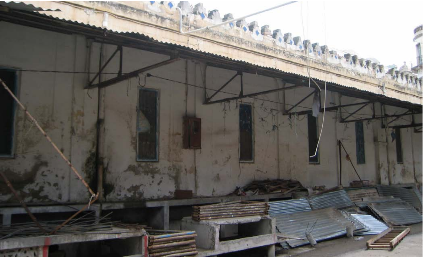
Exterior view of the central building before restoration.
