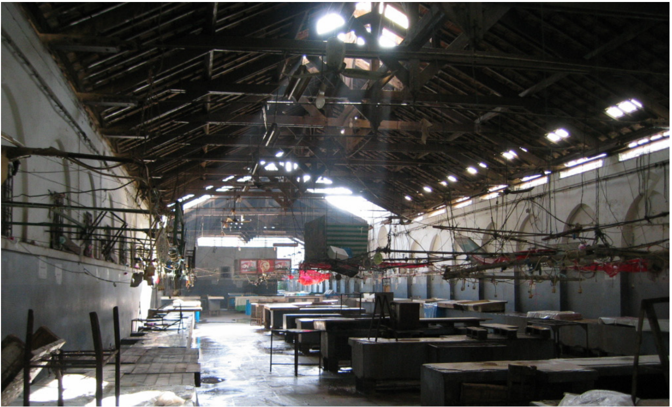
View of the fish market before restoration.
