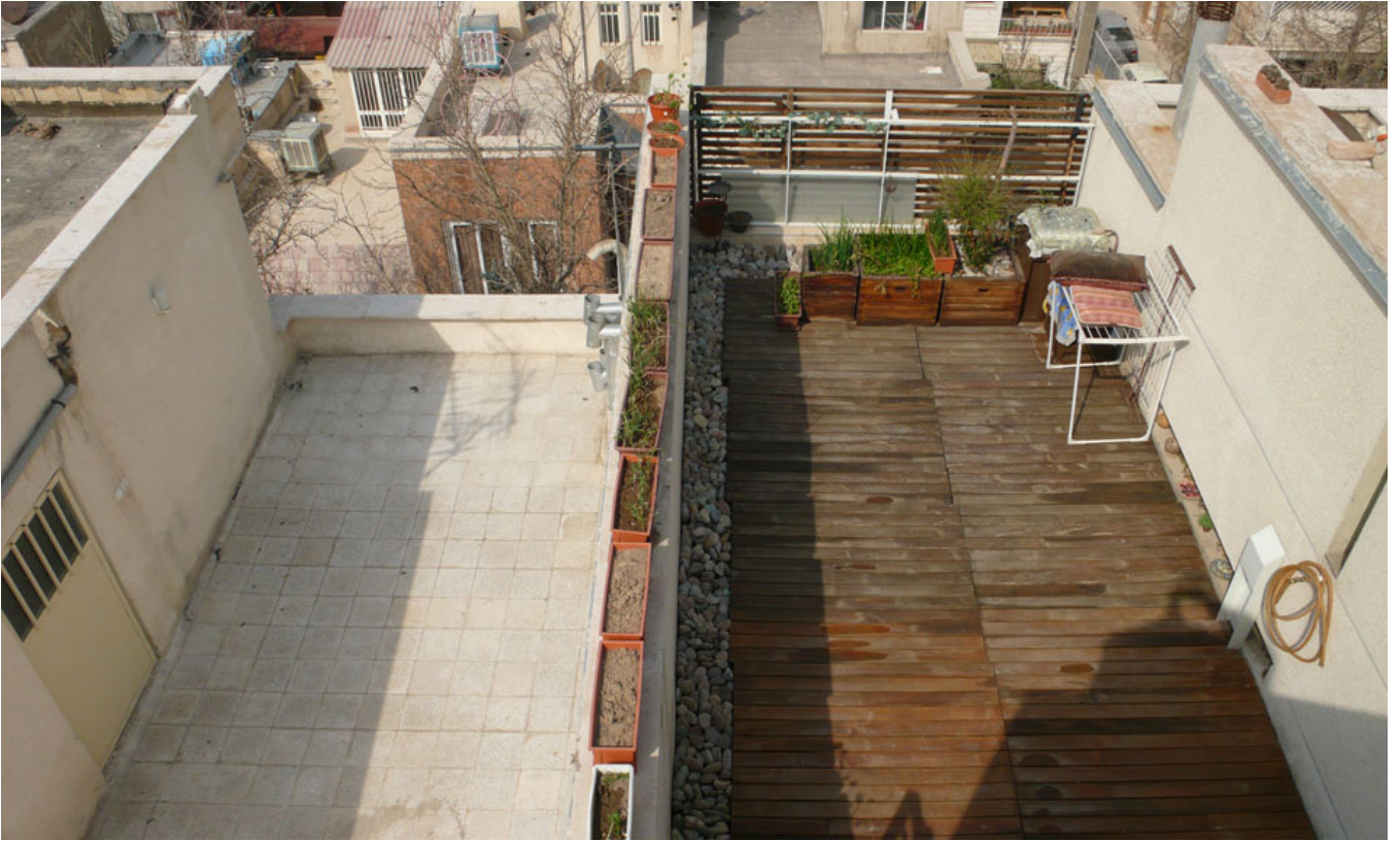
View of the terrace on the fifth floor from the roof.
