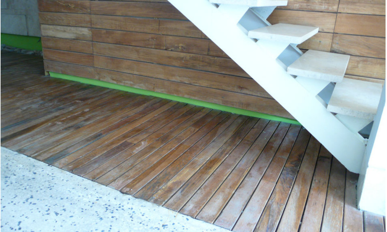
Detail of the wooden deck and stairs.
