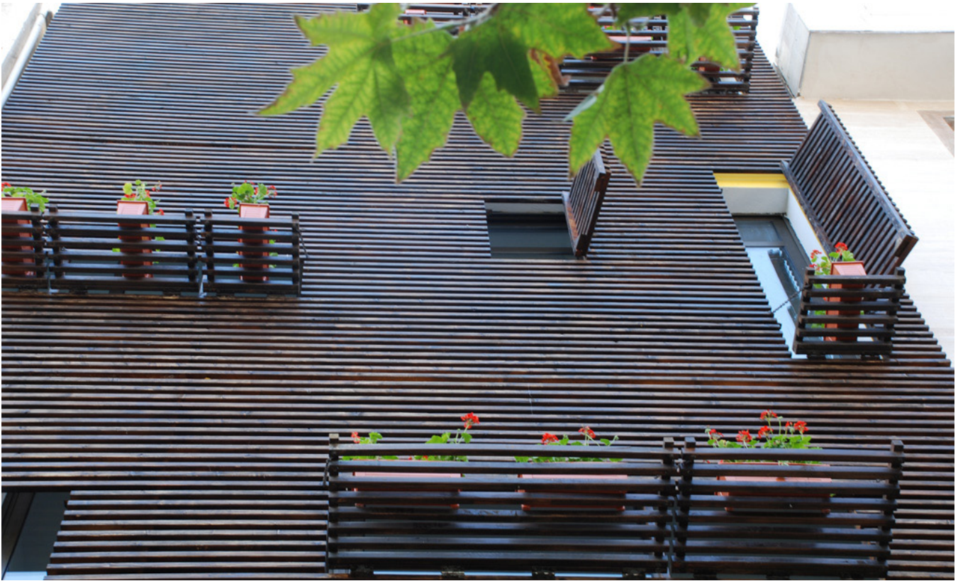
View of the façade, with the panels opened.
