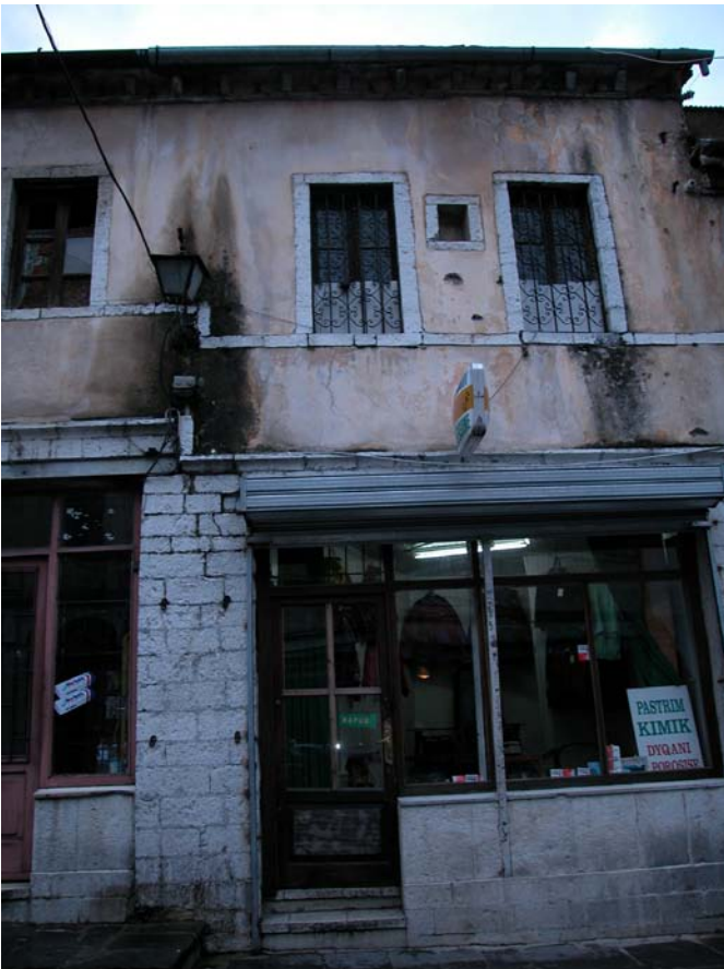
A shop in the bazaar before restoration.
