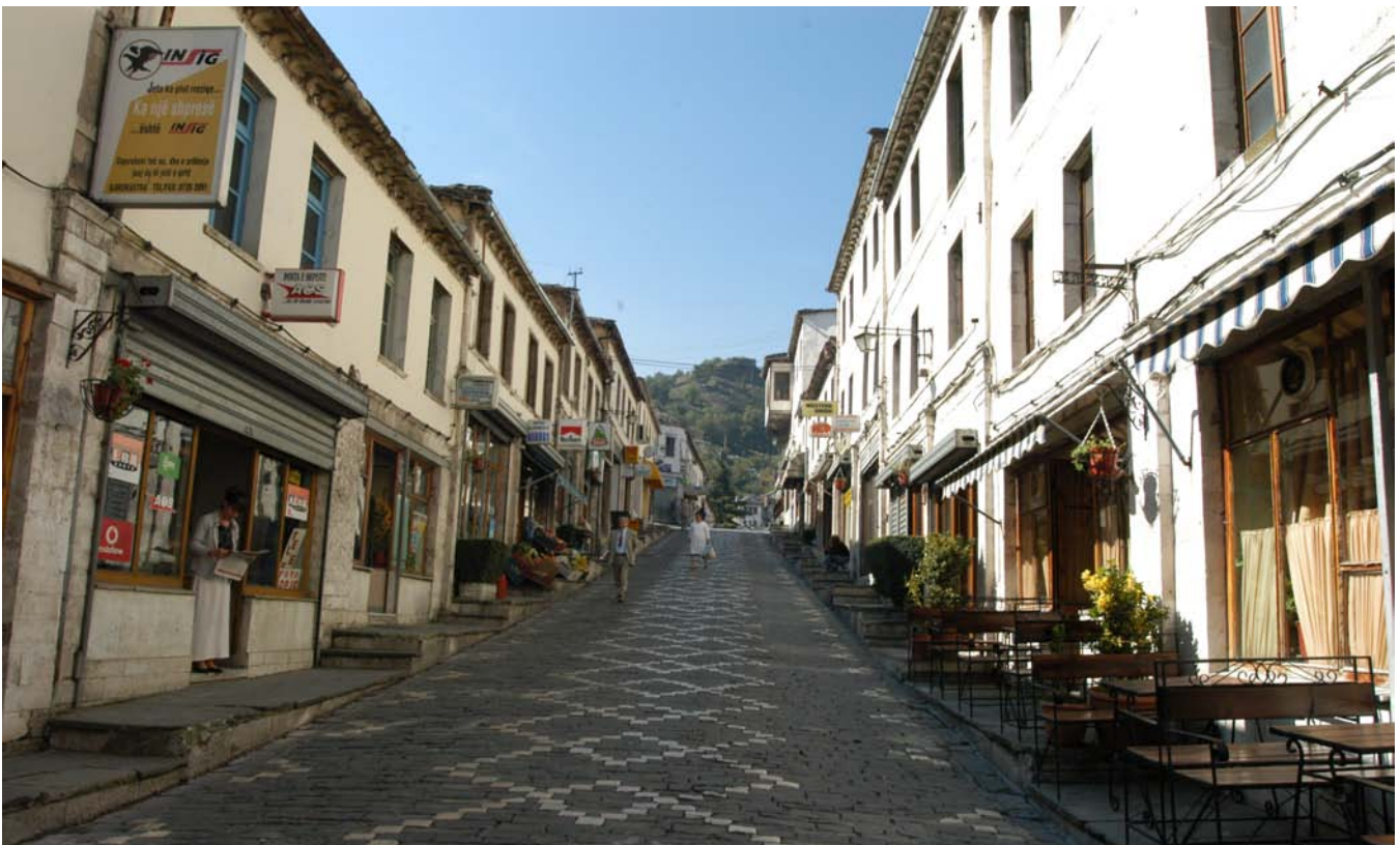
View of the restored bazaar.
