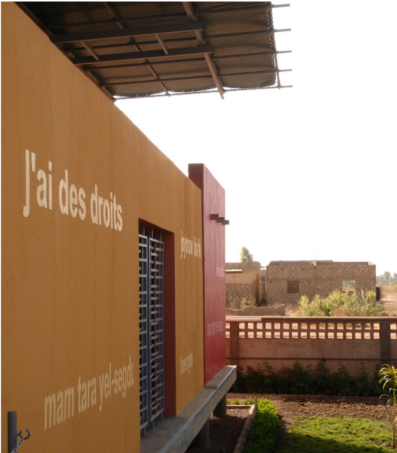
Detail of a wall.
