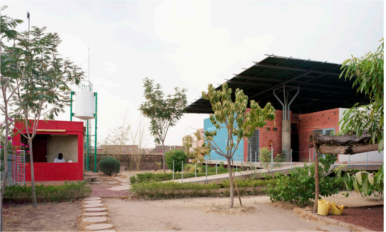
Main entrance and courtyard, with the water tank in the background
