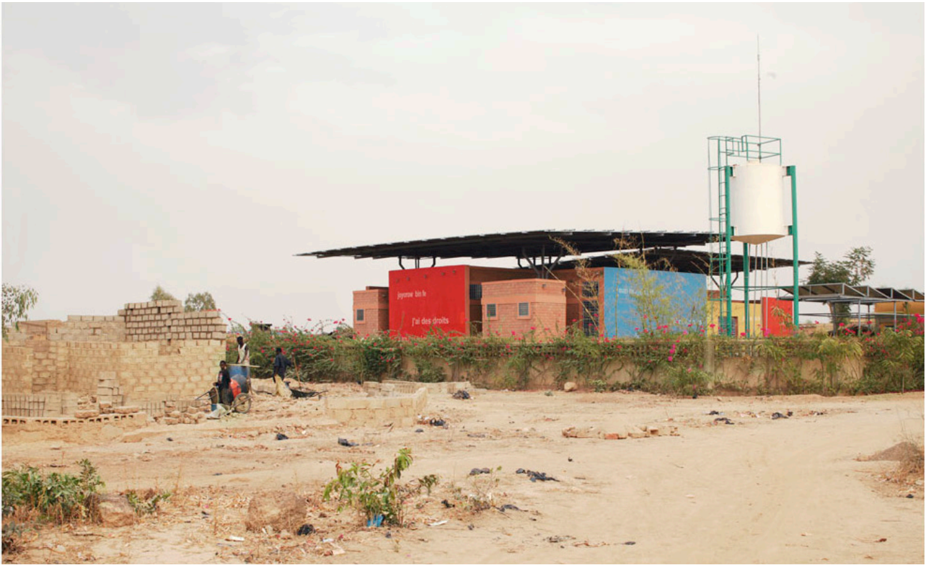
South view of the CBF Womens' Health Centre.
