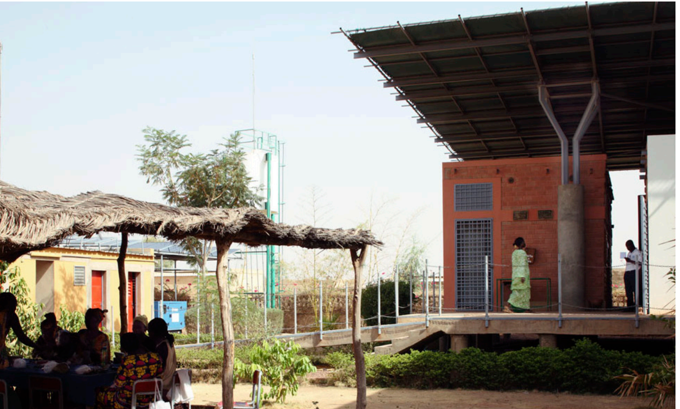
Assembly bungalow in the courtyard. View of the roof, maintained by columns which allows ventilation.
