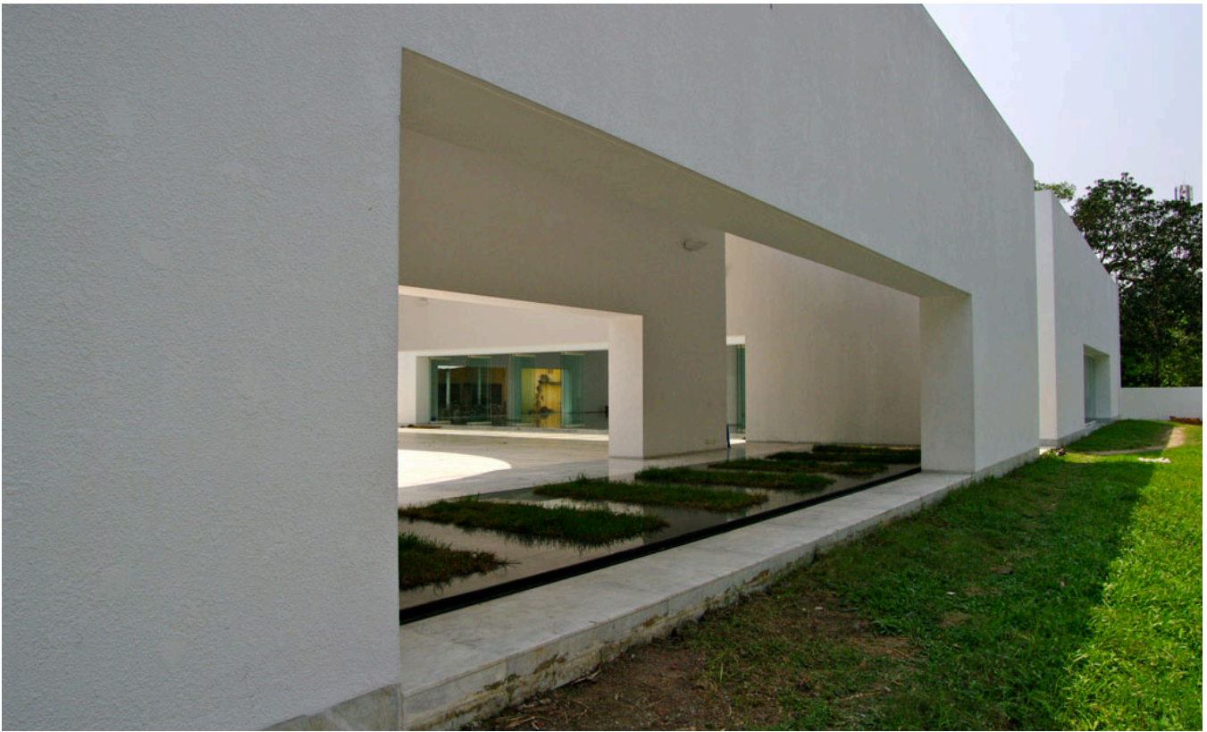
Side view of the front court.
