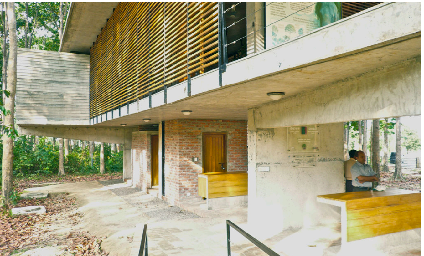
Service blocks at ground floor.
