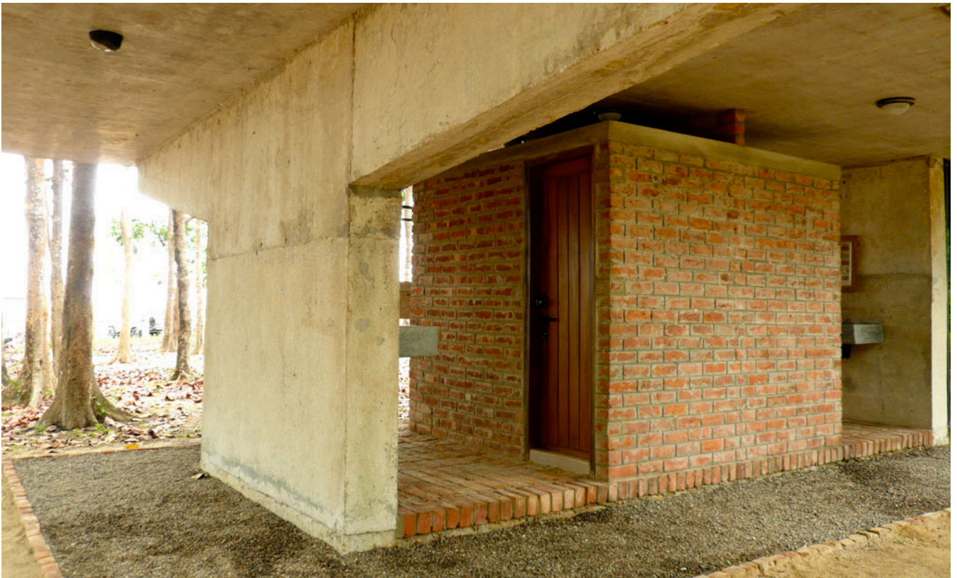
Toilet facilities on the ground floor.
