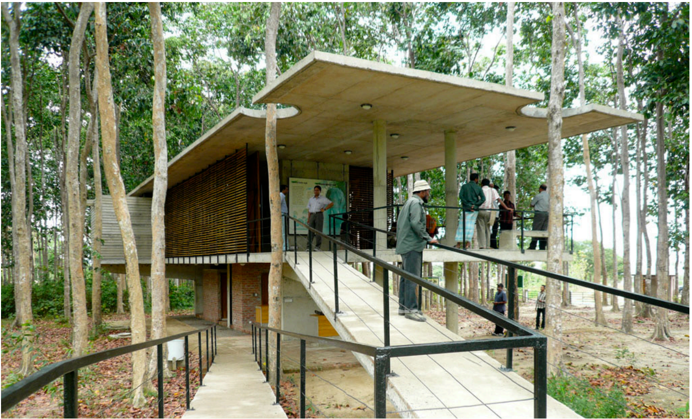
Ramp and pavilion.
