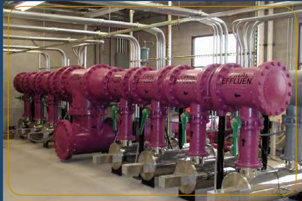
UV disinfection filters eliminates the need for costly and harmful chemical additives.
