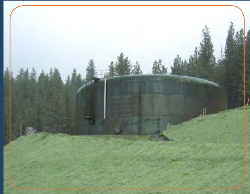
0.65 MG Welded Steel Potable / Fire Water Storage Tank Located at Top of Highest Pressure Zone
