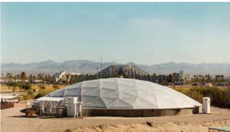
Domestic Water System - Avi Casino - Laughlin, NV
