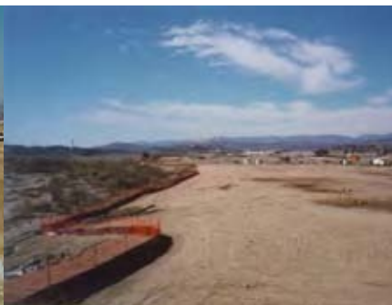
Backfilled soil cement
