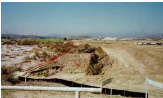
Excavation for soil cement bank protection
