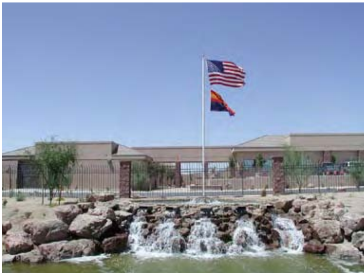
Water Reclamation Facility in Palm Valley - Goodyear, AZ
