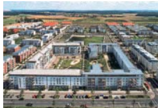
View from the west
