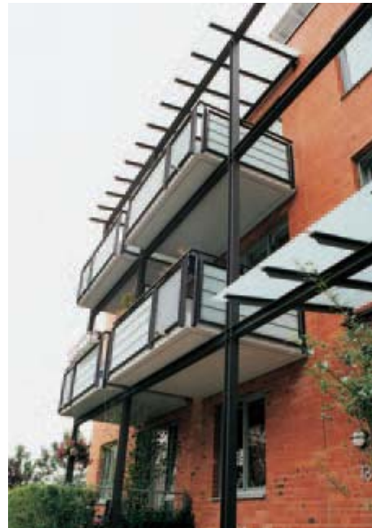
Balcony floors thermally separated from the façade
