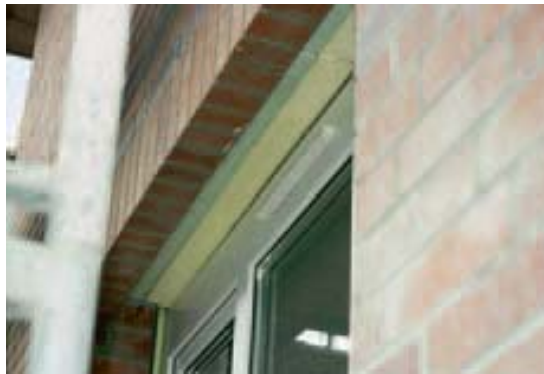
Insulation around a window
