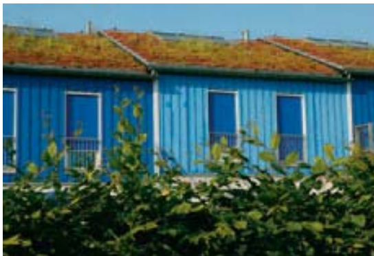
'Lummerland' passive house development
