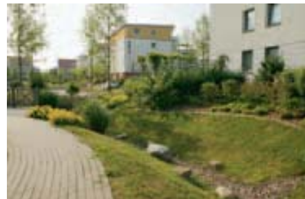
Hollow and trench drainage system
