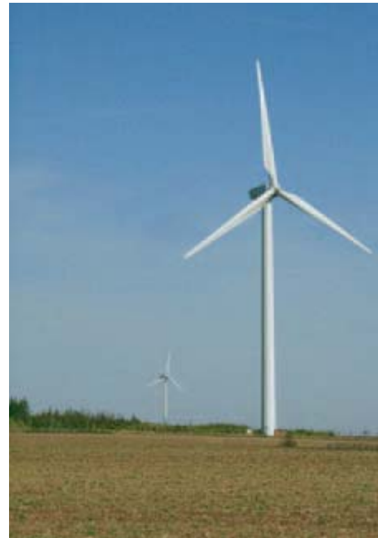
Wind turbine generators in the Kronsberg countryside
