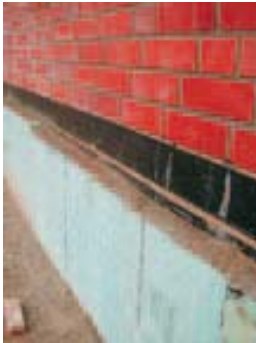
Superinsulating bricks in the base courses
