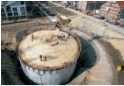
Thermal storage tank under construction
