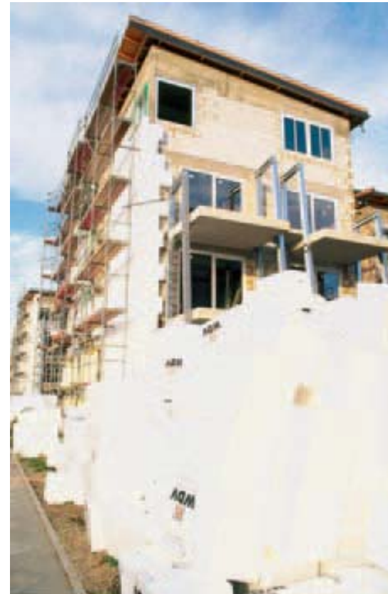
Insulation during construction
