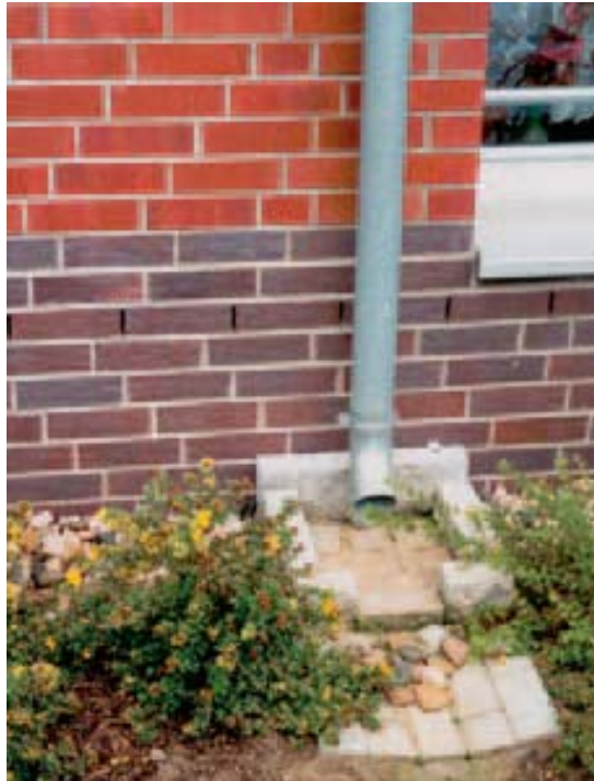
Drainpipes and gullies
