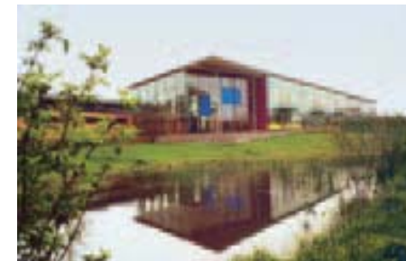
Rainwater retention pond at the primary school
