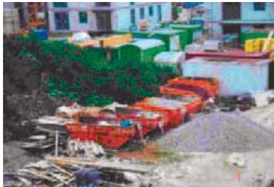
Sorting construction waste
