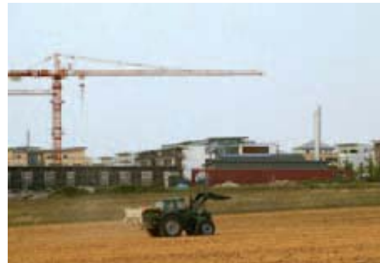
Comprehensive school under construction
